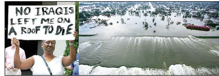
Water Spills Over Collapsed Levy, August 30, 2005
